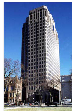
NEW HAVEN OFFICE 157 Church St., 19th Floor New Haven, CT 06510 (203) 427-2906
